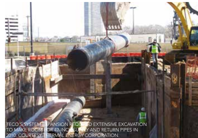
AS PART OF ITS SYSTEM EXPANSION, TECO INSTALLED 42-INCH CHILLED-WATER SUPPLY AND RETURN PIPES IN 2010. COURTESY THERMAL ENERGY CORPORATION.
