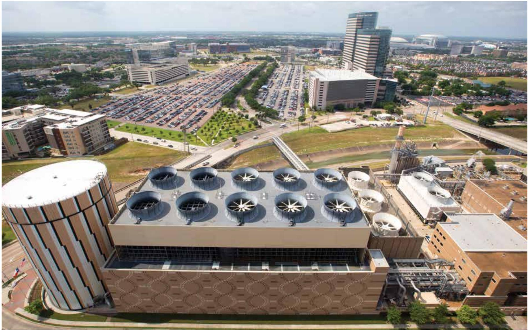
*Located at 1615 Braeswood Blvd., TECO's central plant includes an 8.8 million-gallon thermal storage tank and a modified jet engine that can power a Boeing 747. Facing page: TECO's East Chiller Building contains four 8,000-ton chillers. At 120,000 tons of generating capacity, TECO is the largest district cooling system in North America.*
