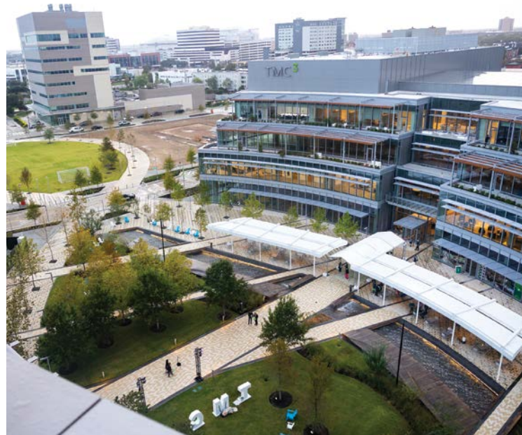
The TMC 3 Collaborative Building is purposefully designed for cohesive and cooperative work between various institutions.
