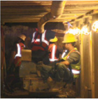
Install 4-inch- x 12-inch-wide oak boards inside 5-ft- x 5-ft-diameter tunnel, adding contiguous ring of boards every foot.
