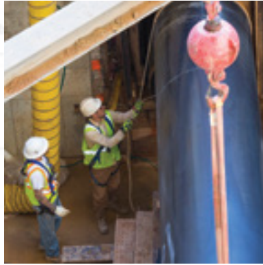
Install TECO's chilled-water and steam pipes inside casings.
