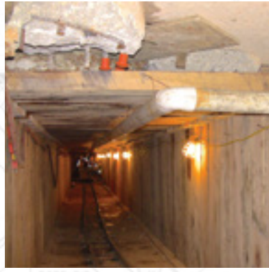
Install 4-inch- x 12-inch-wide oak boards inside 5-ft- x 5-ft-diameter tunnel, adding contiguous ring of boards every foot.
