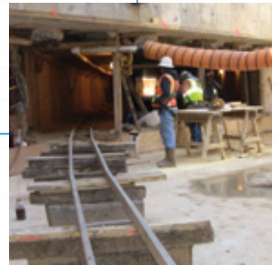
Inject cellular grout to fill void around casing inside each tunnel and seal ends of tunnels.
